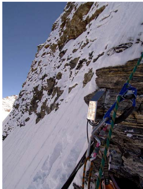
Photo 1: PermaSense "protective shoe" mounted on a little rock spur. In this steel housing, a wireless communication node will be mounted and protected from damage by falling rock or ice (photo: Stephan Gruber)
